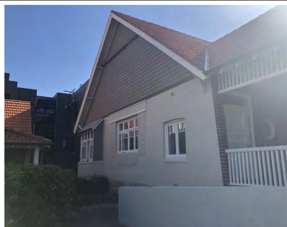
Detail of building showing the detailing and timber shingled gable end. (Source: GML, 2018)
